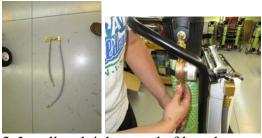
3. Install and tighten end of long hose from Brass quick disconnect kit that is provided to the water meter. Use Teflon tape on threads. Wrench 1 1/8"
