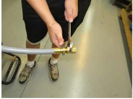
2. Remove fitting from end of hose. The fitting can be thrown away. Wrenches 1" and 7/8
