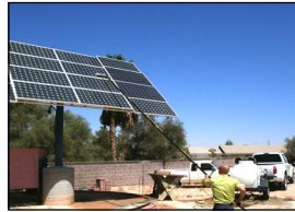
SOLAR PANEL CLEANING
