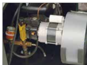
SINGLE PHASE BURNER MOTOR CONNECTED TO FAN AND DIESEL FUEL PUMP
